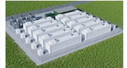
Figure 1. Common site elements and layout for a stationary storage facility. Image not to scale (e.g., larger spacings between containers, and between containers and fence line, are now recommended).
